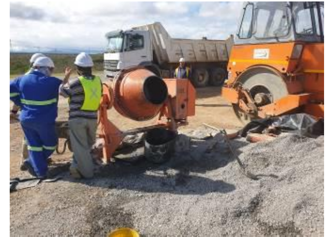
Image 9: Concrete mixing on site.
