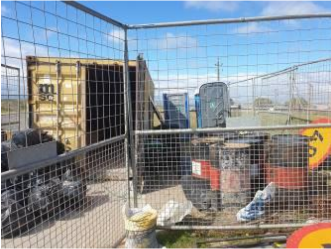
Image 4: Fencing around site camp.
