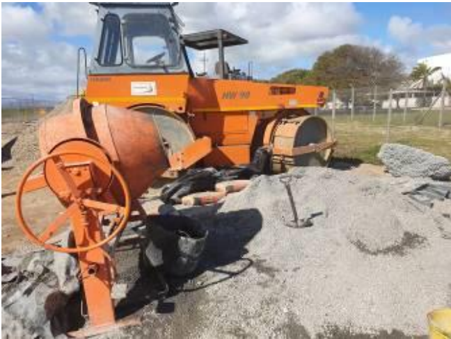
Image 7: Concrete mixing on site.
